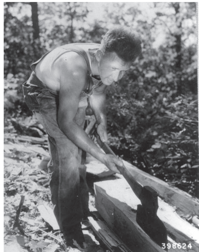
Albert Emily hacking a tie with a broadaxe. U. S. Forest Service photograph courtesy of The State Historical Society of Missouri..
